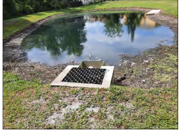
Stormwater Drainage Control Structure
