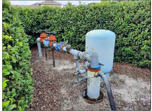
25 HP Well Pump Station
