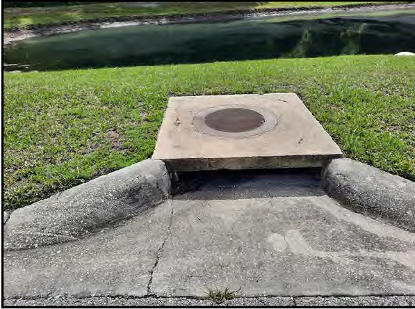
Stormwater Drainage Curb Inlet
