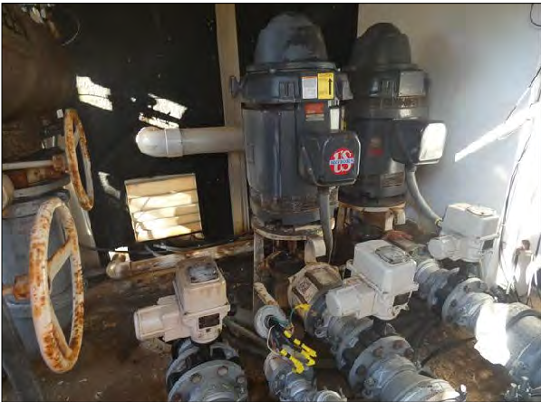
Main Pump Station 60 HP Pumps
