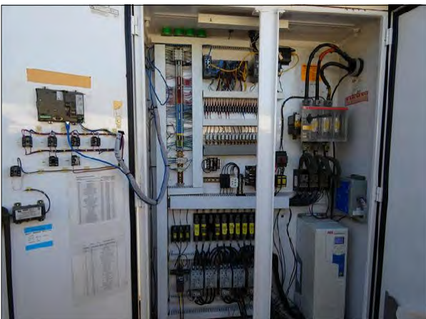
Main Pump Station Controller
